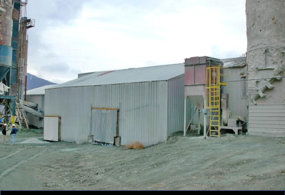
No. 1 granule screening line. Midwestern Multi vibe screens closed circuit with 60 HP hammer mill. Dust collector outside, feed bin on right.
